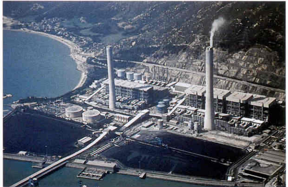
Seven of eight units at China Light & Power were using Wahlco FGC systems when this photo was taken. Plume from eighth unit disappeared when conditioning was activated.
